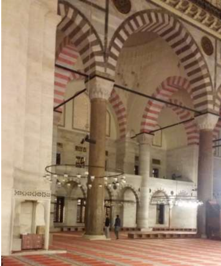
Figure 6. Granite columns supporting the main pillars (Photograph by Author).
